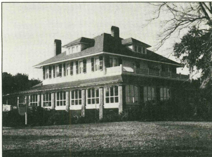
Strachan mansion offers luxury dining, drinking and guestrooms for members of the Haig Point development on Daufuskie Island. The mansion was transported by barge from a plantation on the mainland to provide a gracious setting for social gatherings.
